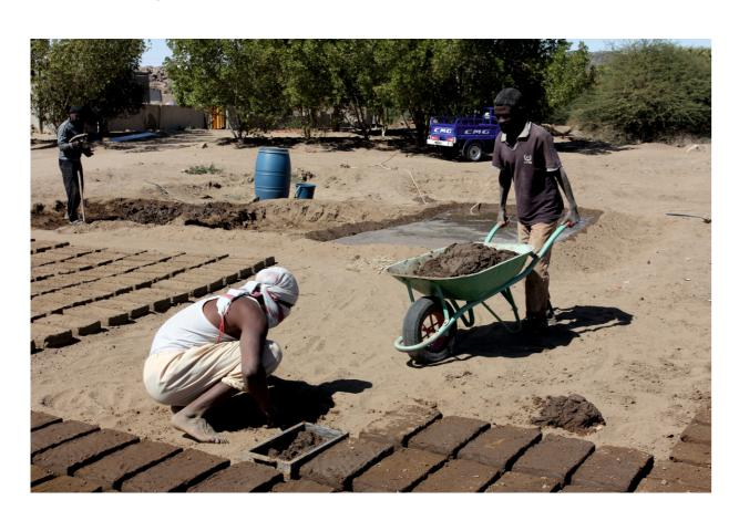
Local builders made mudbricks according to original dimensions, using traditional methods to reinforce and restore the walls.
